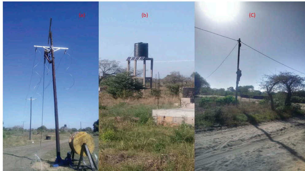
Figure 2. Examples of electrification of rural areas in Mozambique using on-grid system in (a) and (c) by EDM and using an off-grid PV system for water supply by FUNAE (b) (photo by Miguel M. Uamusse).
